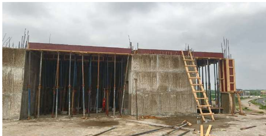
Slab of Lift Shaft Area on terrace floor
